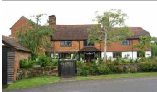
The stone wall in front of Tile House
