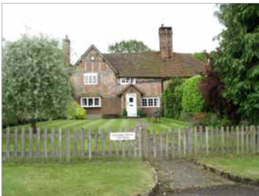
Golden Cross Cottage, Rumbolds Lane
