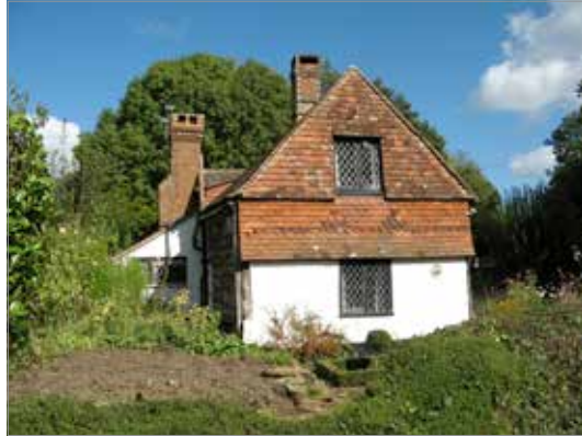
Tile hanging in Loxwood Road
