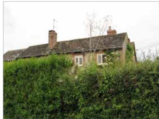
Horsham stone slate roof, and stone-faced elevations, to The Stone House, The Street
